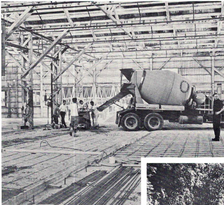
Floor for new press is laid.
