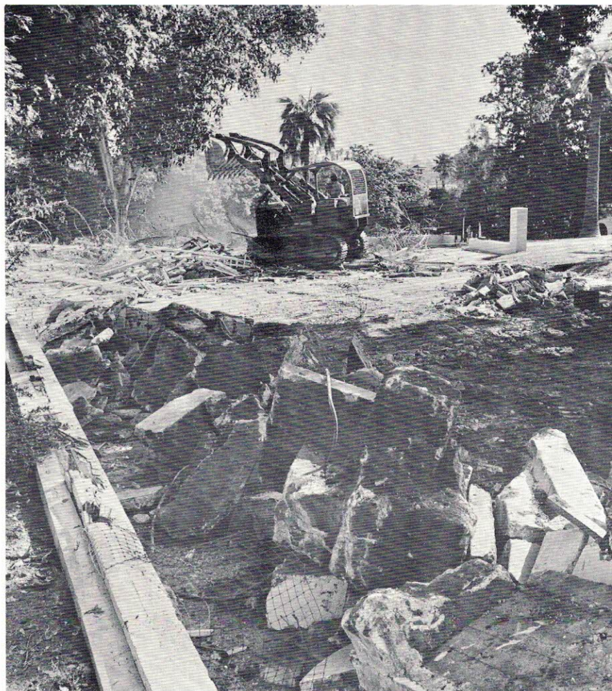
Landscape changes as old tennis courts are ground to rubble.
